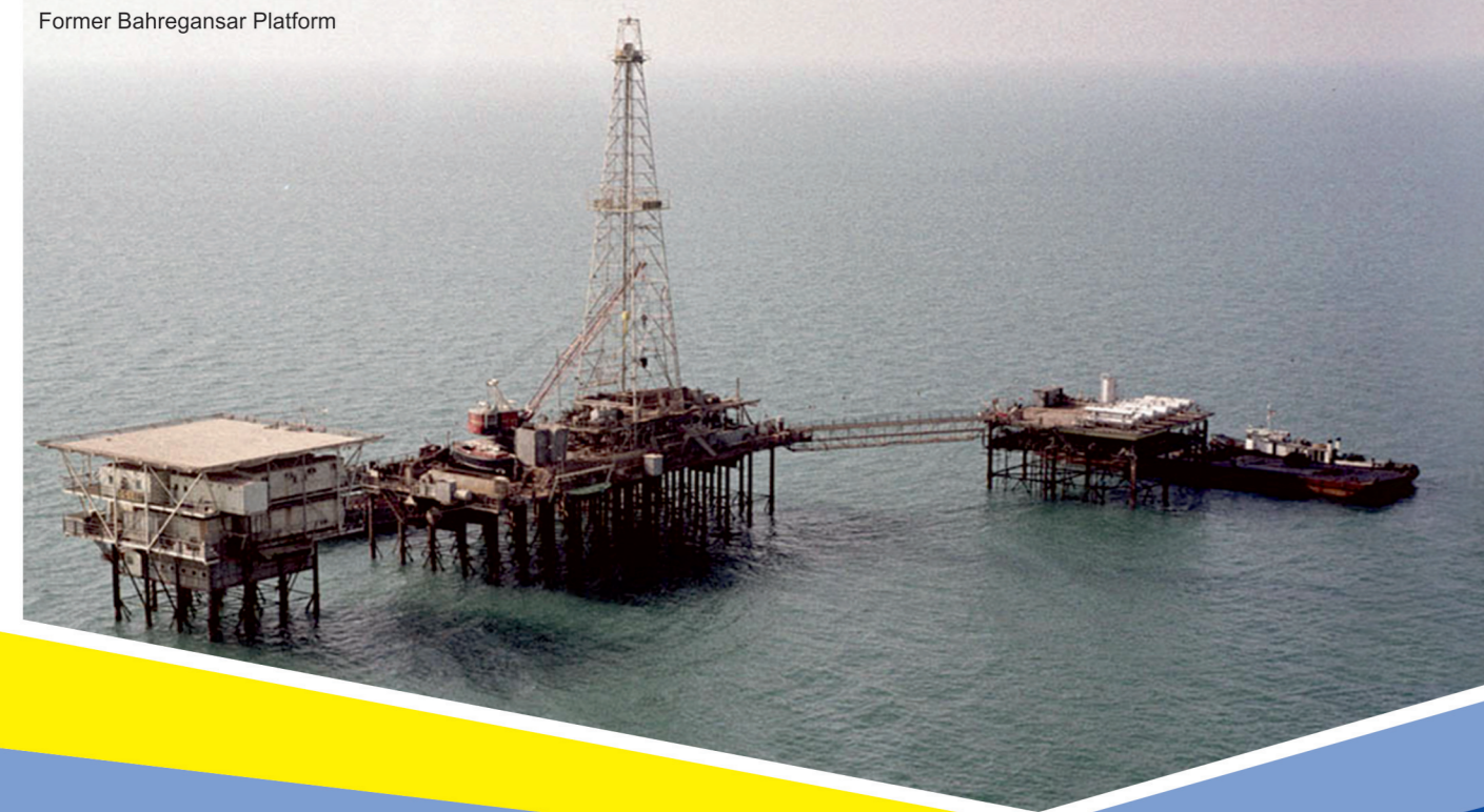
Former Bahregansar Platform
